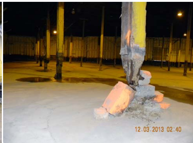
Typical rotted timber columns
